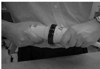
9 Align device and boot indicators and lubricate mouth of boot and rear shoulder of device with soap solution and pull into place.
